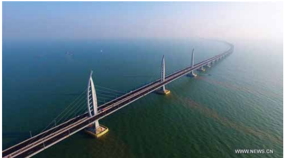
Aerial photo of the Hong Kong-Zhuhai-Macao Bridge on Dec. 27, 2017.
