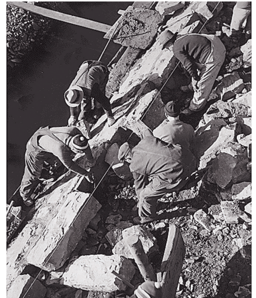
Works Progress Administration (WPA) construction.
