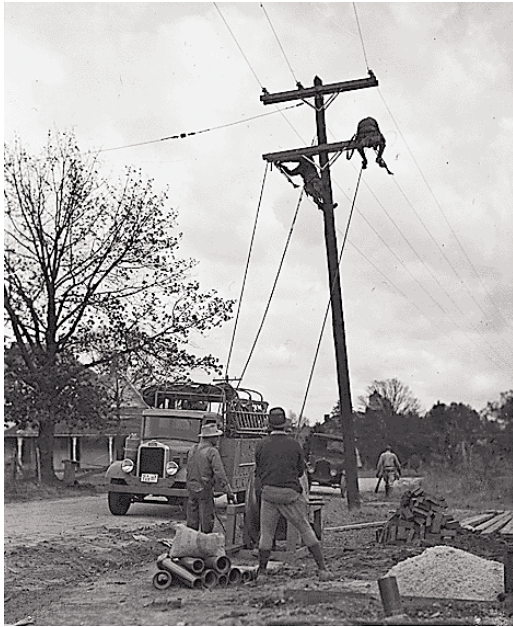
Tennessee Valley Authority (TVA) power line installation, part of Franklin Roosevelt's "New Deal" rural electrification.
