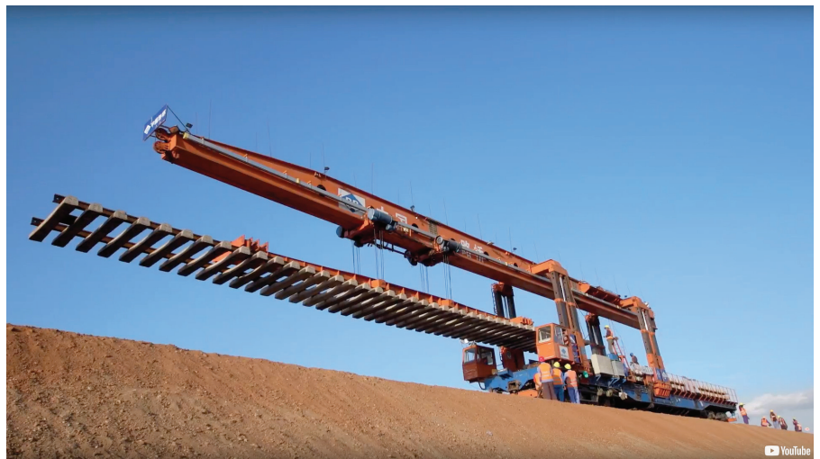
Track-laying machine at work on Mombasa-Nairobi railway.
