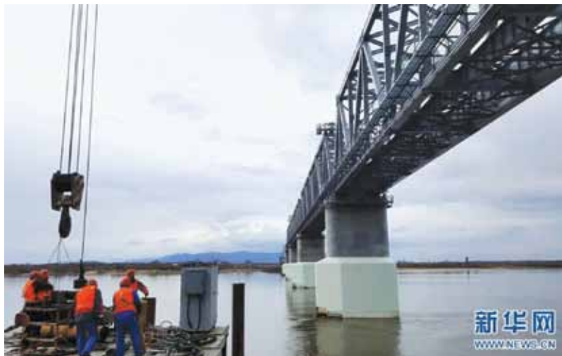
Railroad bridge nears completion, linking Tongjiang City in northeast China’s Heilongjiang Province with Nizhneleninskoye in Russia’s Jewish Autonomous Oblast.
