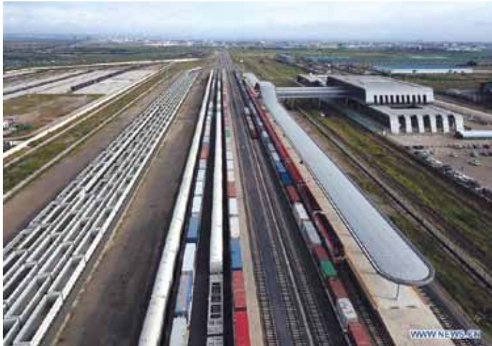
Nairobi terminal of the new Mombasa-Nairobi rail line.
