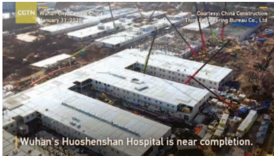
Huoshenshan Hospital nearing completion on January 31, 2020.
