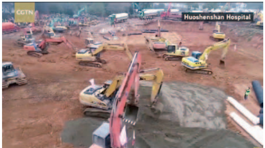
Site preparation begins for Huoshenshan Hospital.
