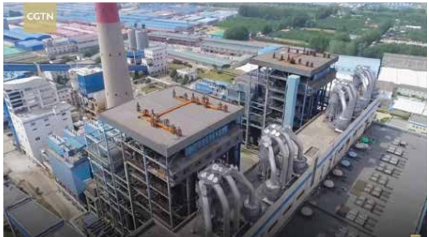
China will optimize its coal production capacity and build advanced coal-fired power plants in line with its development needs. Shown: a low-emissions coal-fired power plant in 2019.
