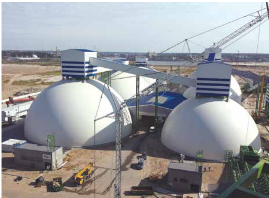
The Riga Fertilizer Terminal in Riga, Latvia, the most modern and safest transshipment terminal in Europe. Each of the four domes can store up to 25,000 tons of fertilizer. September 10, 2013.
