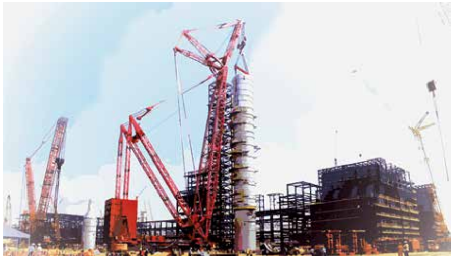
World's largest crude oil distillation column under construction at the Dangote refinery.
