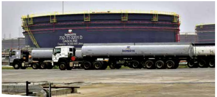
Dangote Industries Limited media page Gasoline tank, capacity 30 million liters, at the Dangote refinery. The refinery is the largest in Africa.
