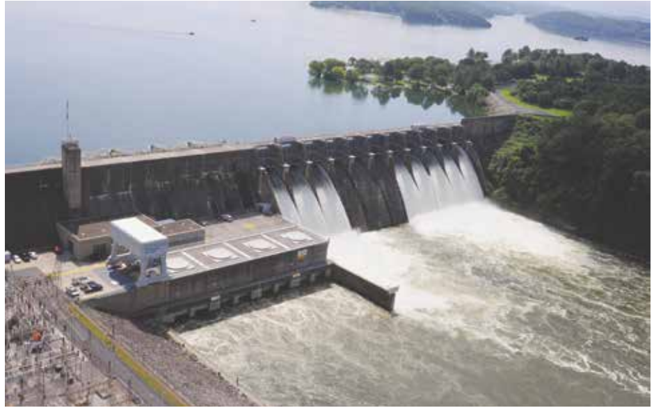
In the early 1940s, the TVA built Douglas Dam in eastern central Tennessee, shown here in a 2013 aerial photograph. During Helene, its reservoir filled to capacity, but performed as designed.
