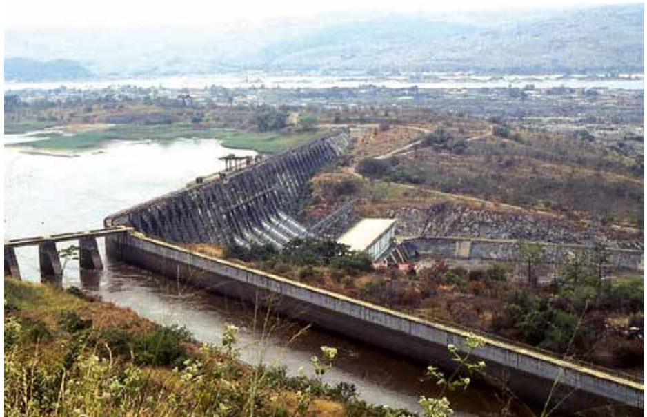
Access to abundant energy is a first step in large-scale economic development. Shown: the Inga I Dam, with the feeding canal for Inga II in the foreground. Construction of six more dams will expand the project's hydroelectric power generation capacity to 40,000 MW, the largest in the world.
