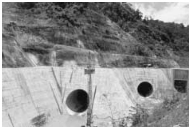
Diversion tunnels have already been drilled in preparation for the dam construction.
