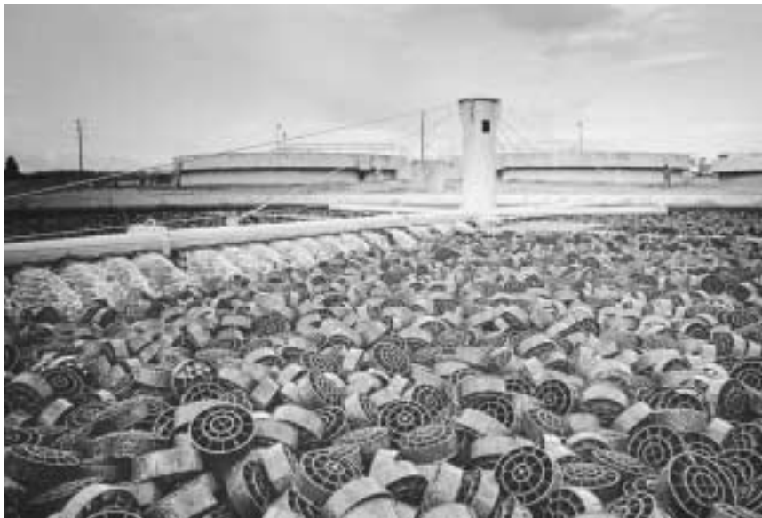
Filtering media of a 15-year-old sewage treatment plant in Virginia. Vast amounts of U.S. water treatment and runoff infrastructure is four to ten times that age, and breaking down; our national water-treatment “debt” is near $1 trillion in replacement costs.
