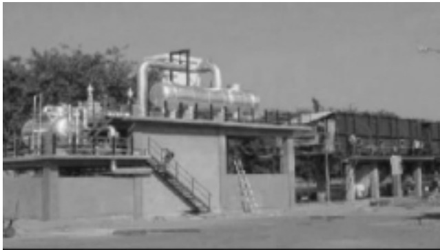
This 4,500-cubic-meters-per-day Multi-Stage Flash desalination plant is under construction, inside the nuclear facility at Kalpakkam, in Tamil Nadu state.
