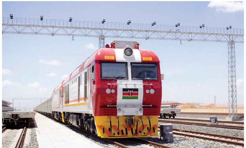
The Standard Gauge Railway connecting Kenya’s capital Nairobi to the port city Mombasa, built by China, opened in 2017—the largest infrastructure project in Kenya since independence in 1963.
