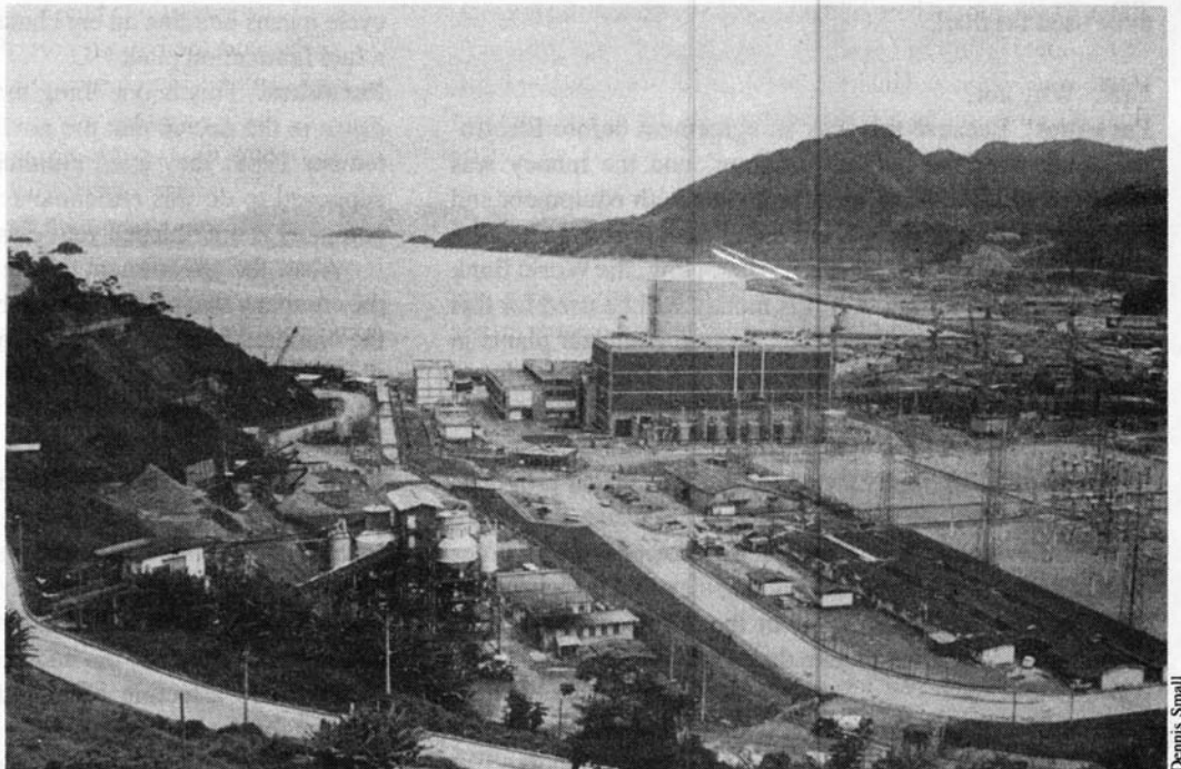
Brazil's first nuclear plant, the Angra 1, which went into operation in 1984.
