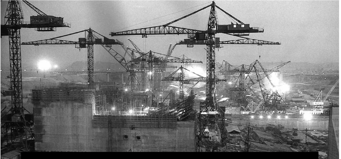
The construction of the Gezhou Dam in China.
