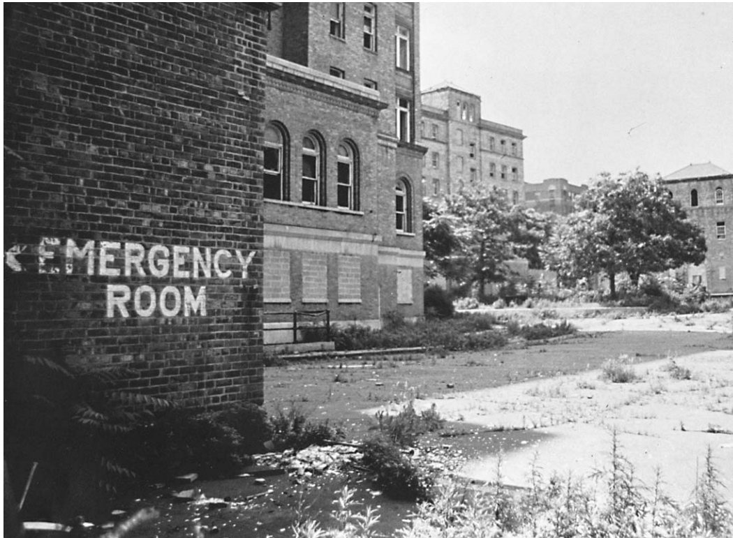
The collapse of urban infrastructure and health care are vital issues which were ignored by both leading Presidential candidates. Here, what used to be a hospital in New York's South Bronx.
