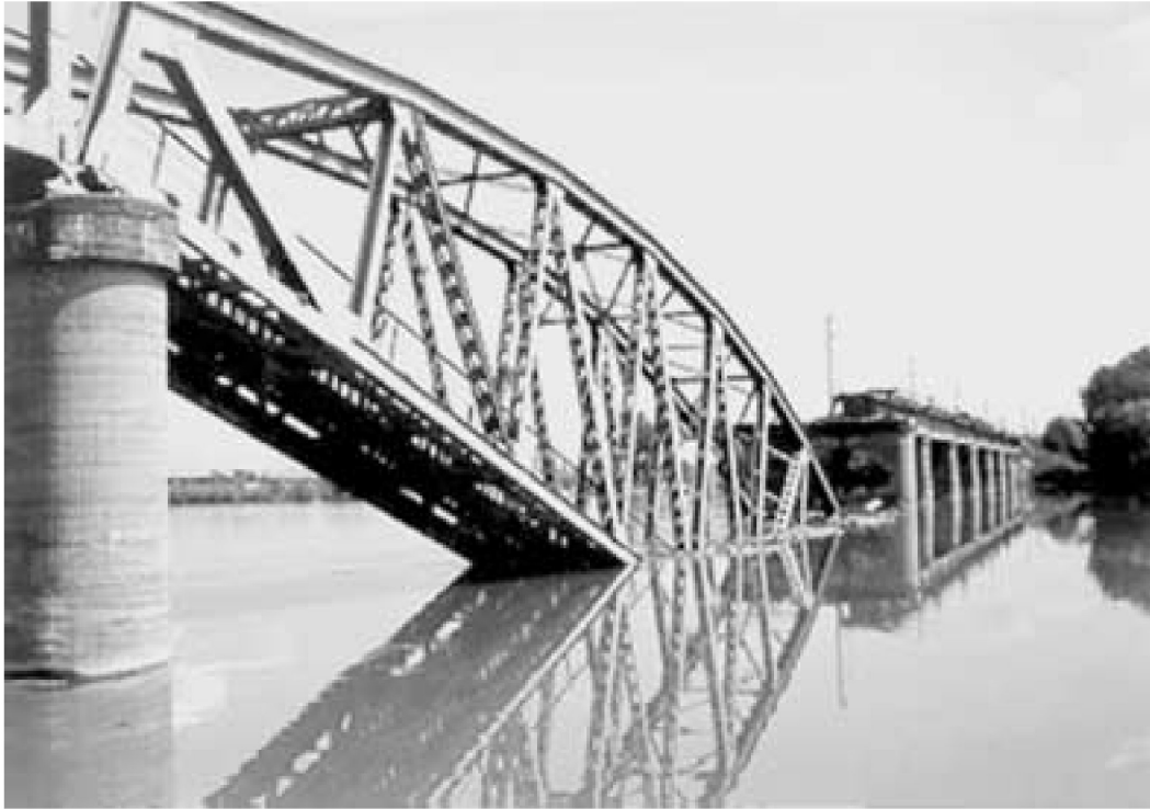
The Ostruznica railway bridge in Belgrade, destroyed by the U.S.-British bombing of Yugoslavia in May 1999. "We say to those who are duped into admiring the utopians: 'Soldier, could you rebuild what you just blew up?'"
