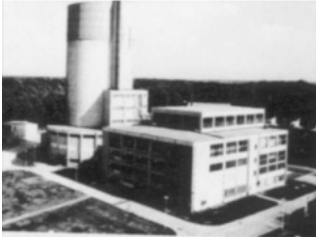
The AVR experimental pebble bed reactor in Jülich, Germany, came on line in 1967 and operated successfully for 22 years. It demonstrated many safety effects of the high-temperature reactor. One test with the AVR showed that in a total sudden shutdown, the plant cools down and the fuel pebbles remain intact.
