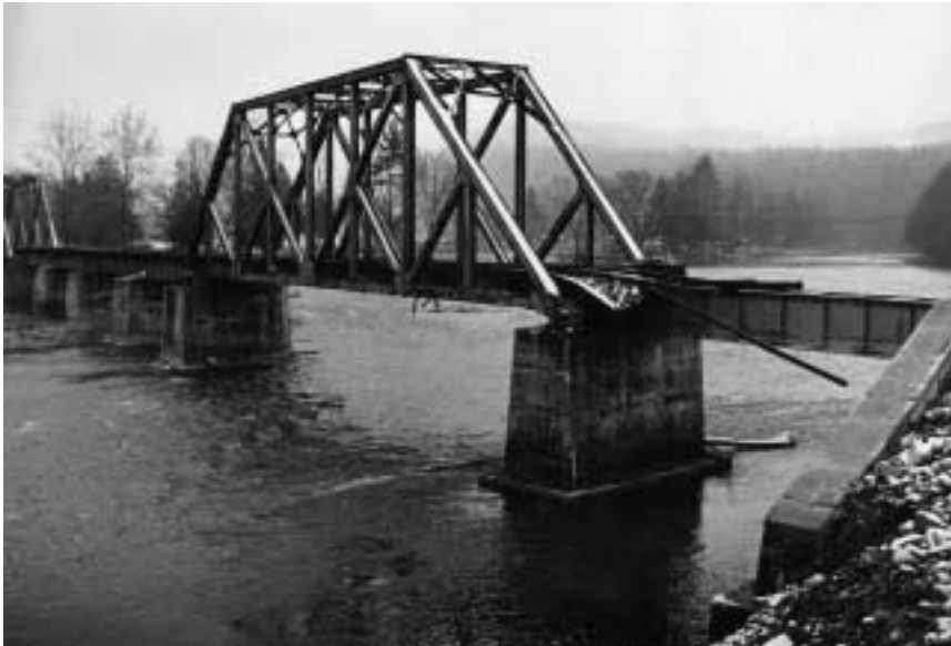
The general, foolish presumption of the apologists for “fiscal austerity” plundering of wealth being depleted, “is that if the bridge did not collapse immediately once the maintenance is discontinued, the result is a cost-saving to be merrily added to the ‘bottom line.’ ” Here: the result of fiscal austerity in West Virginia.
