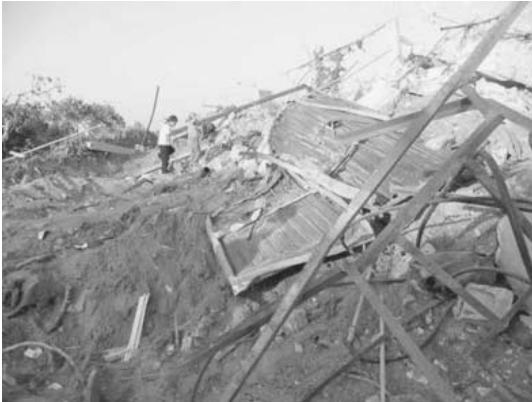
Beit Hanoun on the West Bank, in late May 2003, after demolition by Israeli Defense Forces armored vehicles. While “accepting” the Road Map, Sharon has his forces continuing incursions, killings, and demolitions throughout the occupied territories.
