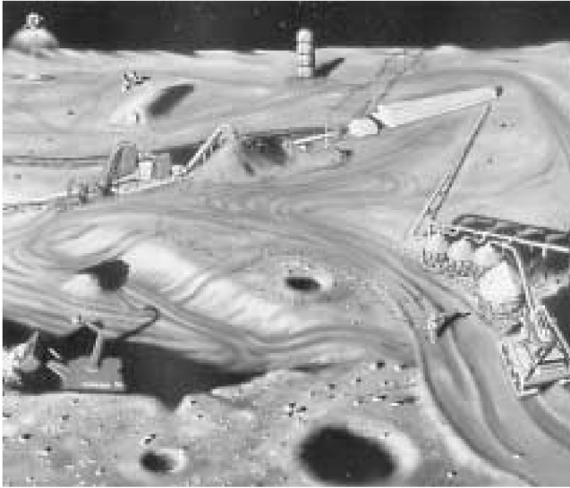
The process of lunar industrialization prepared the way for colonizing Mars. Here, a lunar resource processing pilot plant, designed to develop the technologies used for collection, analysis, and both mechanical and electrochemical separation of lunar surface resources. It produces materials needed for life support and propulsion (such as oxygen); and fabrication and construction of structural elements.
