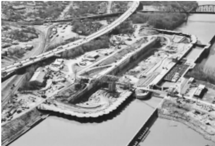
Shown in the photo at left looking down the Ohio River at Louisville, the Army Corps of Engineers' long-stalled plan to replace the old 600-foot McAlpine Lock (at right center of the photo), with a modern 1,200-foot lock (excavation, center), was delayed so long by funding cuts, that metal fatigue in the old lock's wall forced emergency closure of the Ohio River since mid-August. On the right is a schematic of the new lock, this time looking upstream. Nationally, neglect of water infrastructure is "close to catastrophe," says the Army Corps' director.
