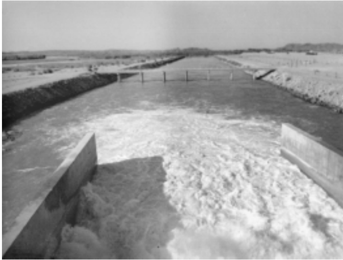
The 80-mile All-American Canal, looking from the overflow section of the Imperial Dam on the Colorado River. These waterworks were built during FDR's New Deal. The Canal, completed in 1940, began carrying water in 1942, to eventually irrigate some 500,000 acres in the Imperial Valley, through a system of 2,900 miles of laterals. Ditches carry off surplus water to the Alamo River. The Imperial Dam, completed in 1938, was the second on the Colorado, after the Hoover Dam. The Canal is among water and power installations run by the Imperial Irrigation District, set up in 1911 to administer power and water to a service area today covering 6,471 square miles in the Valley.
