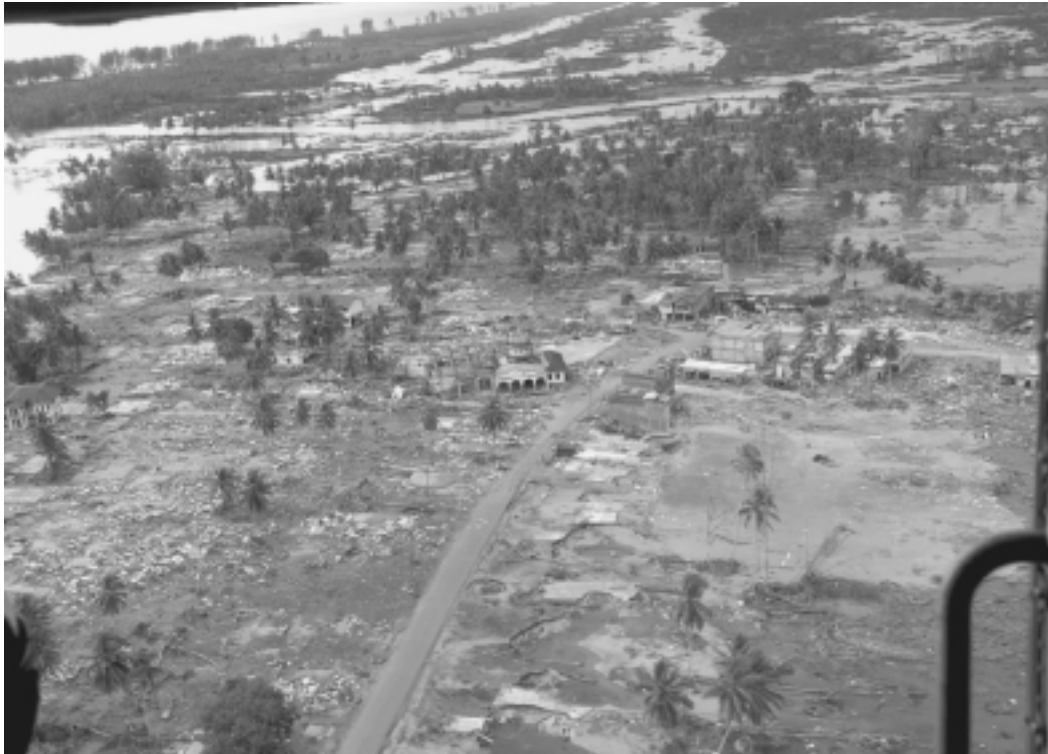
Banda Aceh, Indonesia, one of the regions worst-hit by the Dec. 26 tsunami. Germany has proposed a debt moratorium for the devastated nations. Equally essential is to bring the infrastructure of the region into the 21st Century—rather than focussing on restoring the fragile tourism “industry.”
