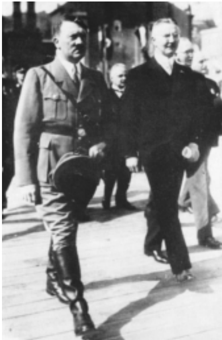
Hjalmar Schacht with Hitler in 1934, at the laying of the foundation stone for the new Reichsbank building.
