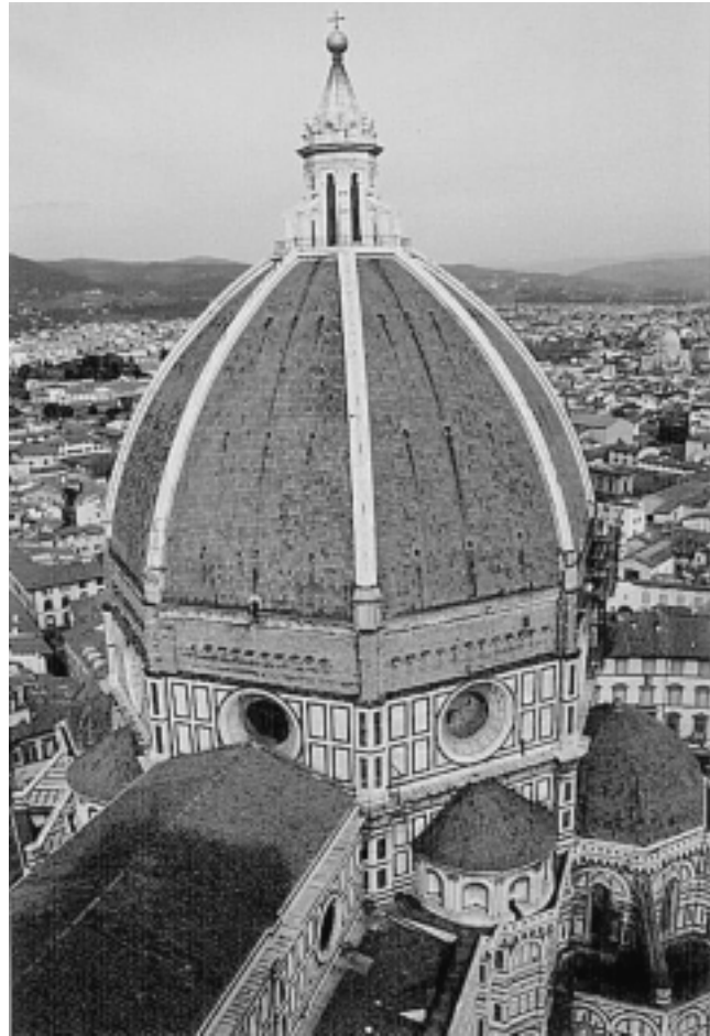
Brunelleschi's dome on the Cathedral of Florence was built in the 15th Century, one of the high points of the Renaissance. The Venetians vowed to destroy what had been achieved at the ecumenical Council of Florence which took place there in 1438-39.
