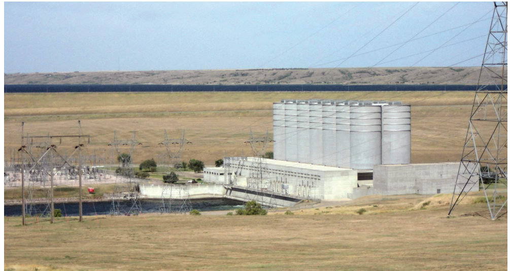
The Oahe Powerhouse, a hydroelectric plant at the Oahe Dam, near Pierre, S.D.
