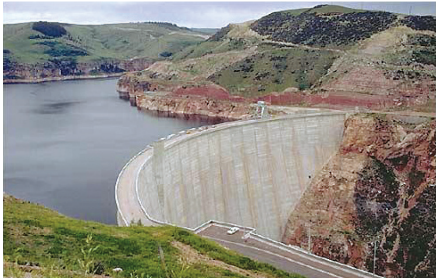
The Bureau of Reclamation’s Yellowtail Dam across Bighorn Canyon in southeastern Montana. This is the largest concrete dam in the Missouri River System.
