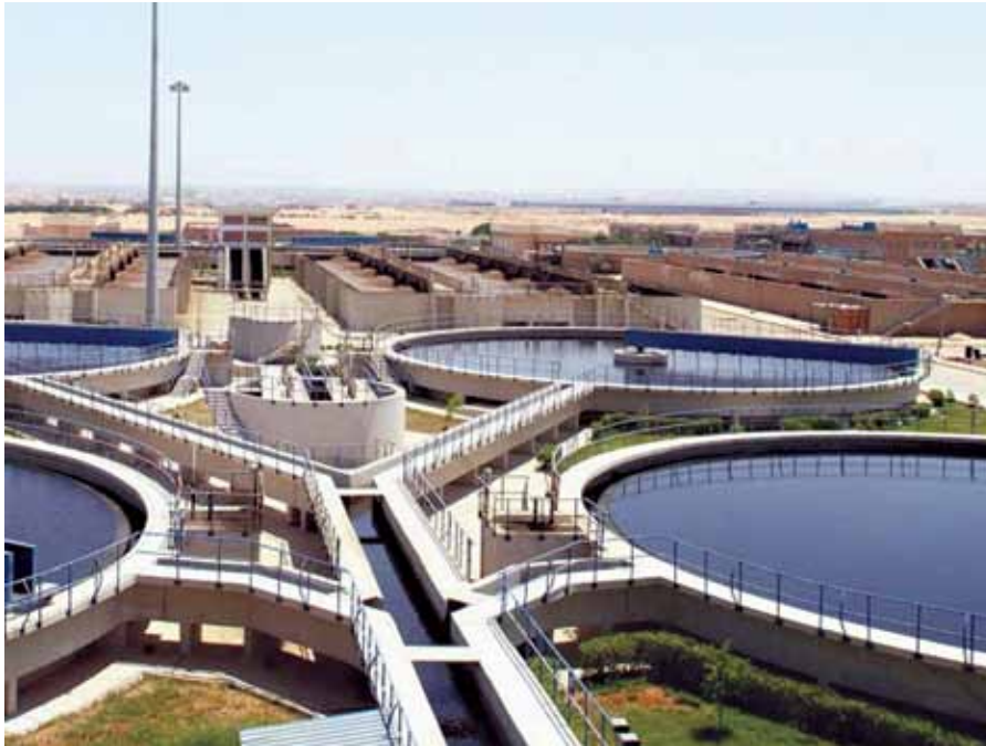
The key three sectors of infrastructure, without which, neither agriculture, nor industry could develop are: energy, water, and transportation. Shown: the El-Sheikh Zayed water-treatment plant, Sheikh Zayed City, Egypt.
