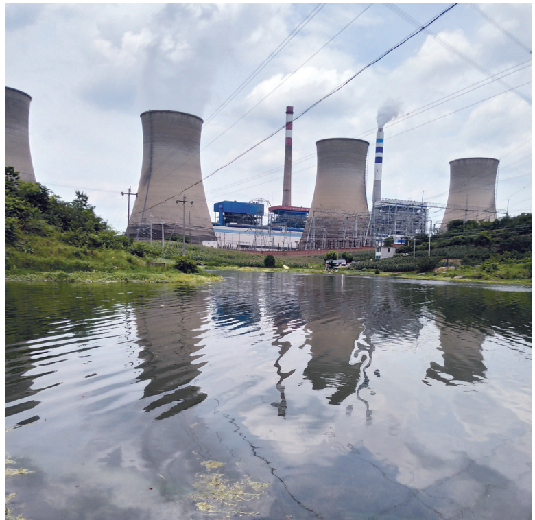
The Qianxi Power Station, a coal-fired power plant near Gantang, Guizhou Province, China.
