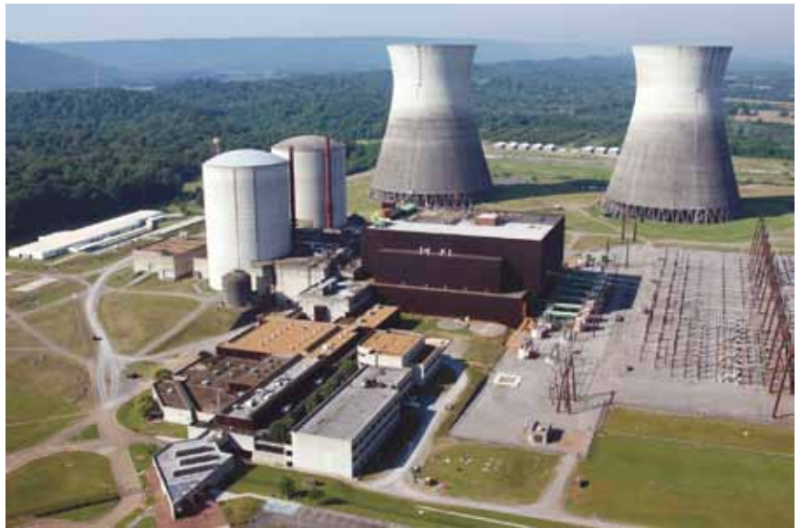
The Bellefonte Nuclear Generating Station in Hollywood, Alabama.
