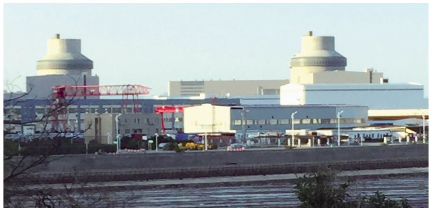
Sanmen Nuclear Power Station, located in Zhejiang, China.
